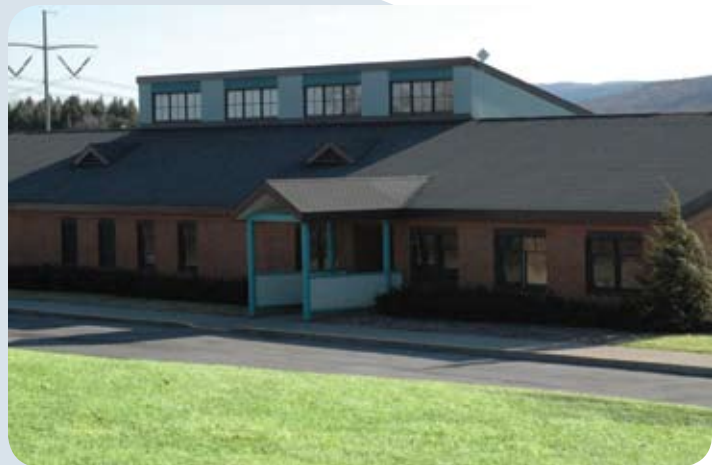
View of Schenectady ARC's Princetown Ridge located in the Town of Princetown.
